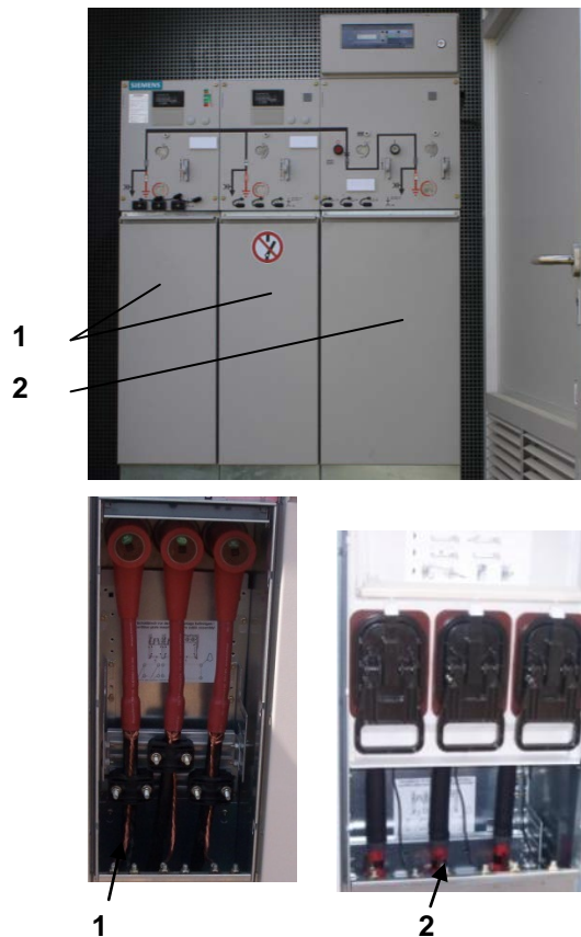
Fig. 19 - Medium-voltage system (example)
