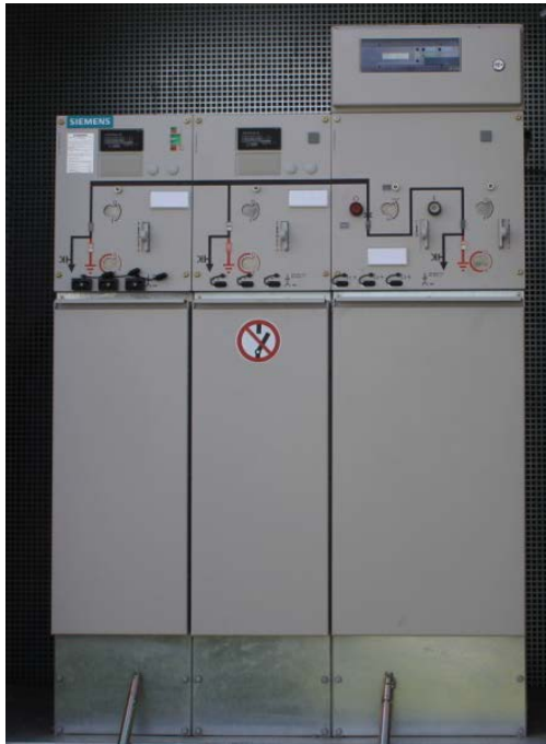
Fig. 10 - Medium-voltage system (example)
