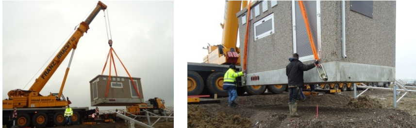
Fig. 14 - Installing the container station
