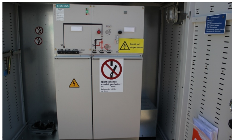
Figure 8 - MV switchgear (example)
